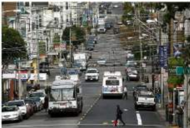
Figure 14 View of the trolleybus overhead contact line network 26 .
